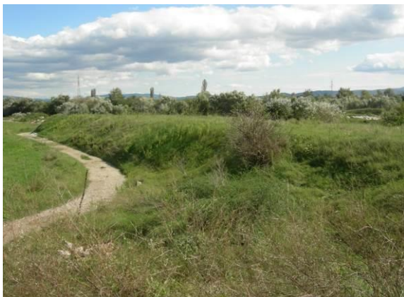
Embankment on the left bank of Vardar river
