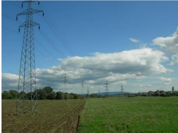
View of the location from the railroad with the power line
