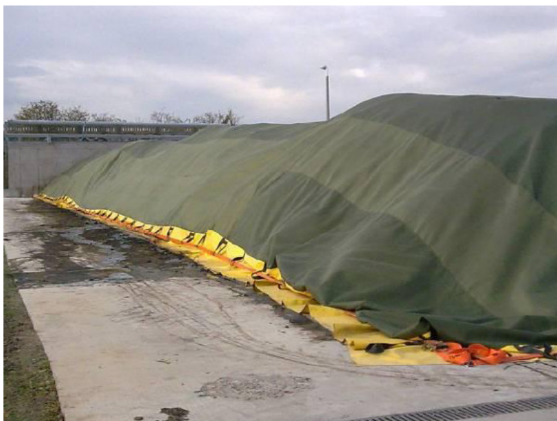
Figure 3-86: a) outdoor windrow composting with heap covered with membrane for protection and odour confinement
