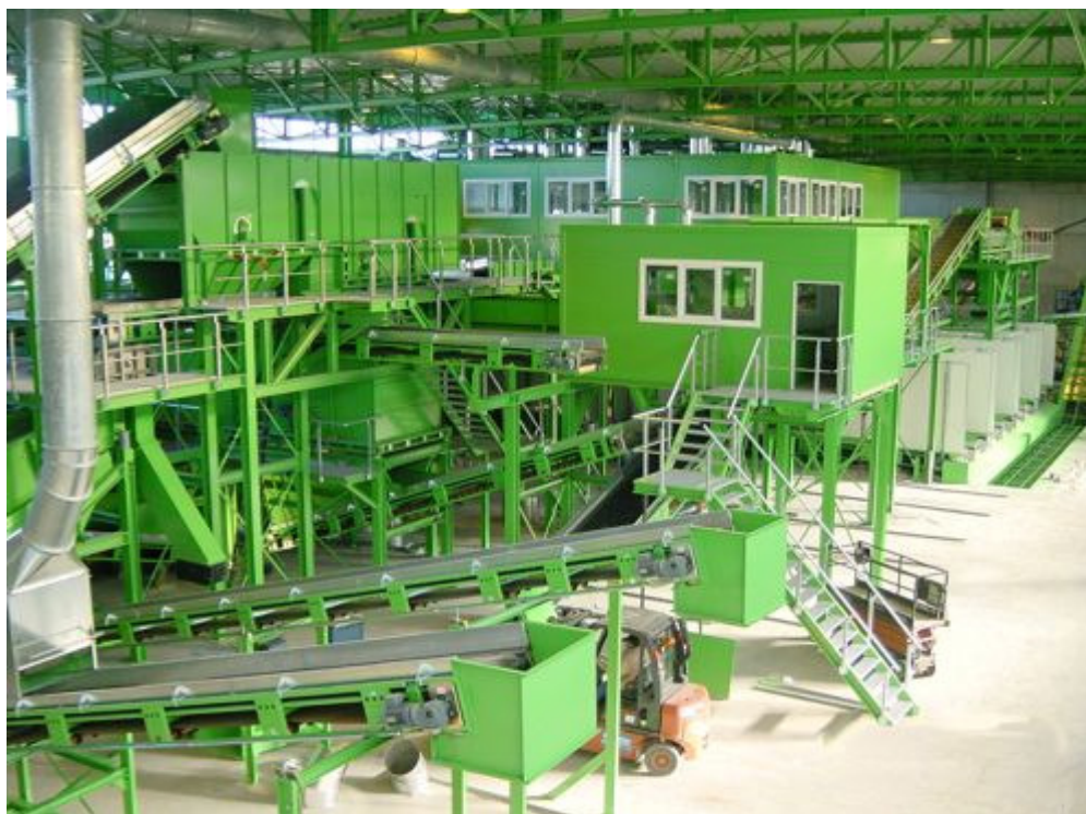
Figure 3-78: MBT plant interior
