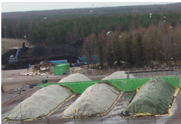
Figure 3-74: Aerated covered heaps (open air area)
