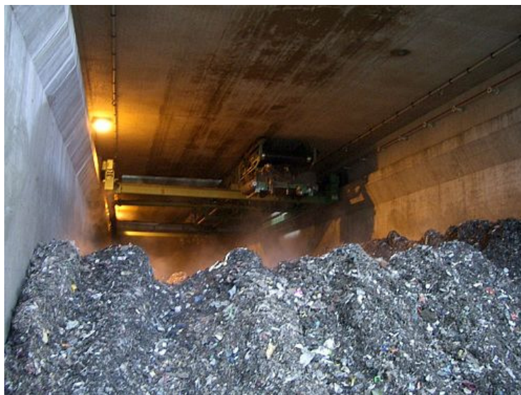
Figure 3-80: MBT composting tunnel
