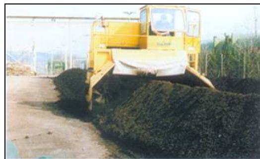
Figure 3-71: Turned windrows compacting system (Open Area)
