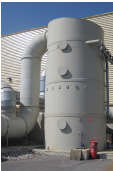
Figure 3-88: a) scrubber and b) biofilter with filling material pending to install
