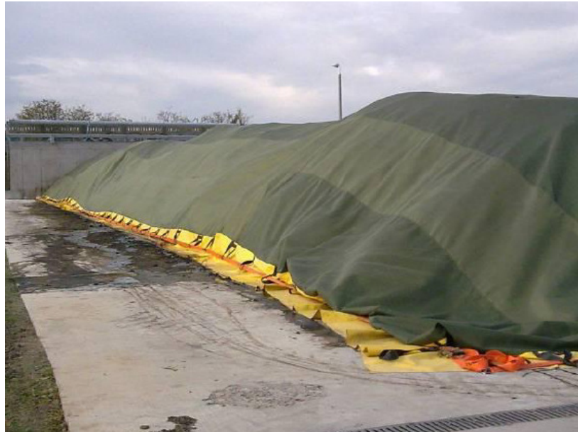
Figure 3-88: Outdoor windrow composting with heap covered with membrane for protection and odour confinement
