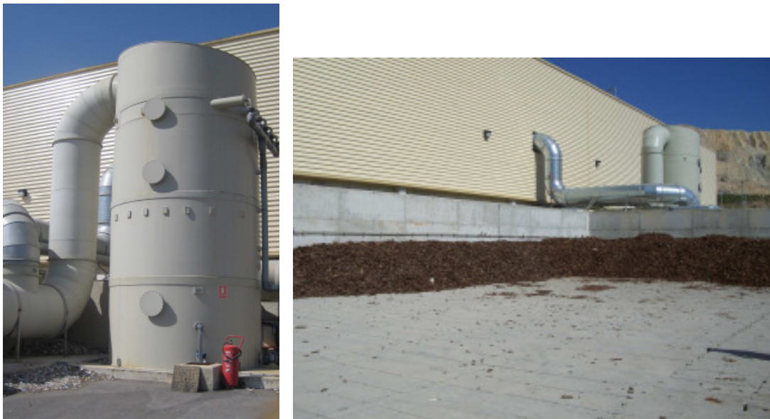
Figure 3-90: a) scrubber and b) biofilter with filling material pending to install
