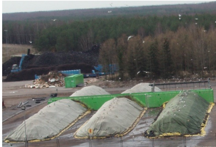
Figure 3-76: Aerated covered heaps (open air area)
