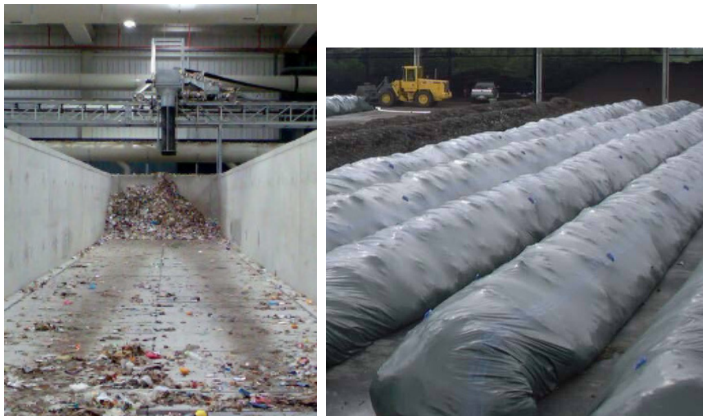
Figure 3-87: a) composting in tunnel (lanes) with perforated aeration floor, b) composting in bags
