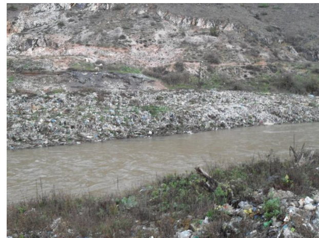
Figure 4 Landfill in Kicevo
