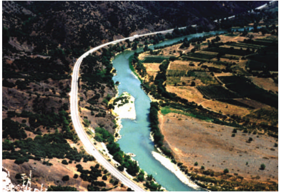
Figure 124. The highway from Demir Kapiya to Gevgeliya (Photo: Lj. Melovski)
