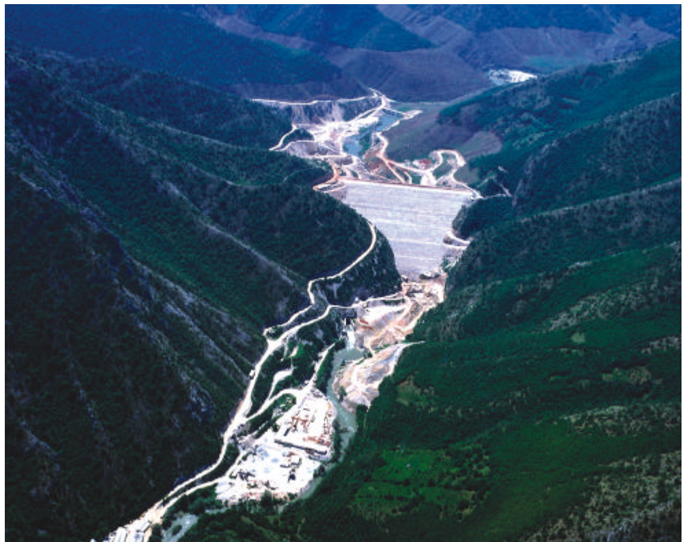
Figure 121. Kozyak Dam (in construction) (Photo: M. Dzingo)
