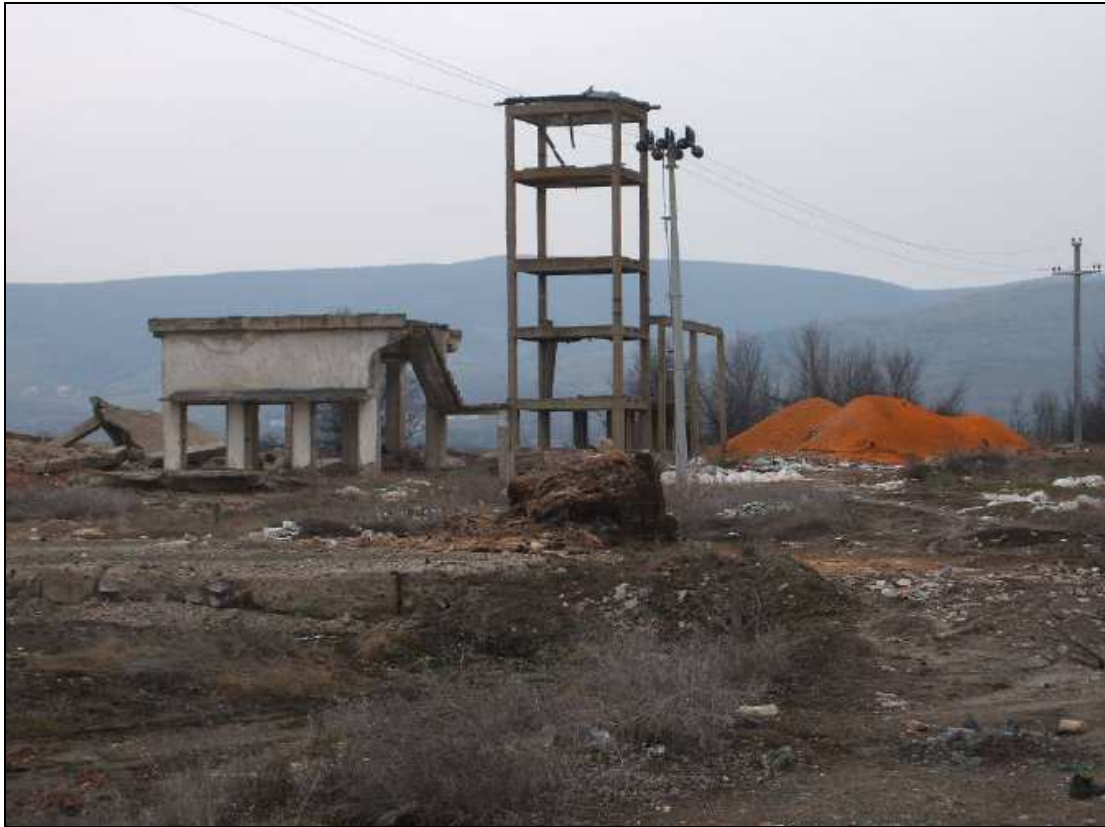
Photo 2.13 – Roasting/smelting facilities – plant ruins
