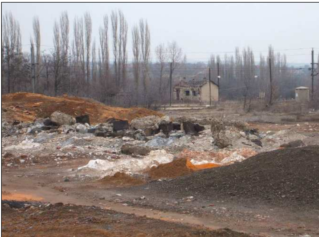
Photo 2.14 – Roasting/smelting facilities – open storage yard
