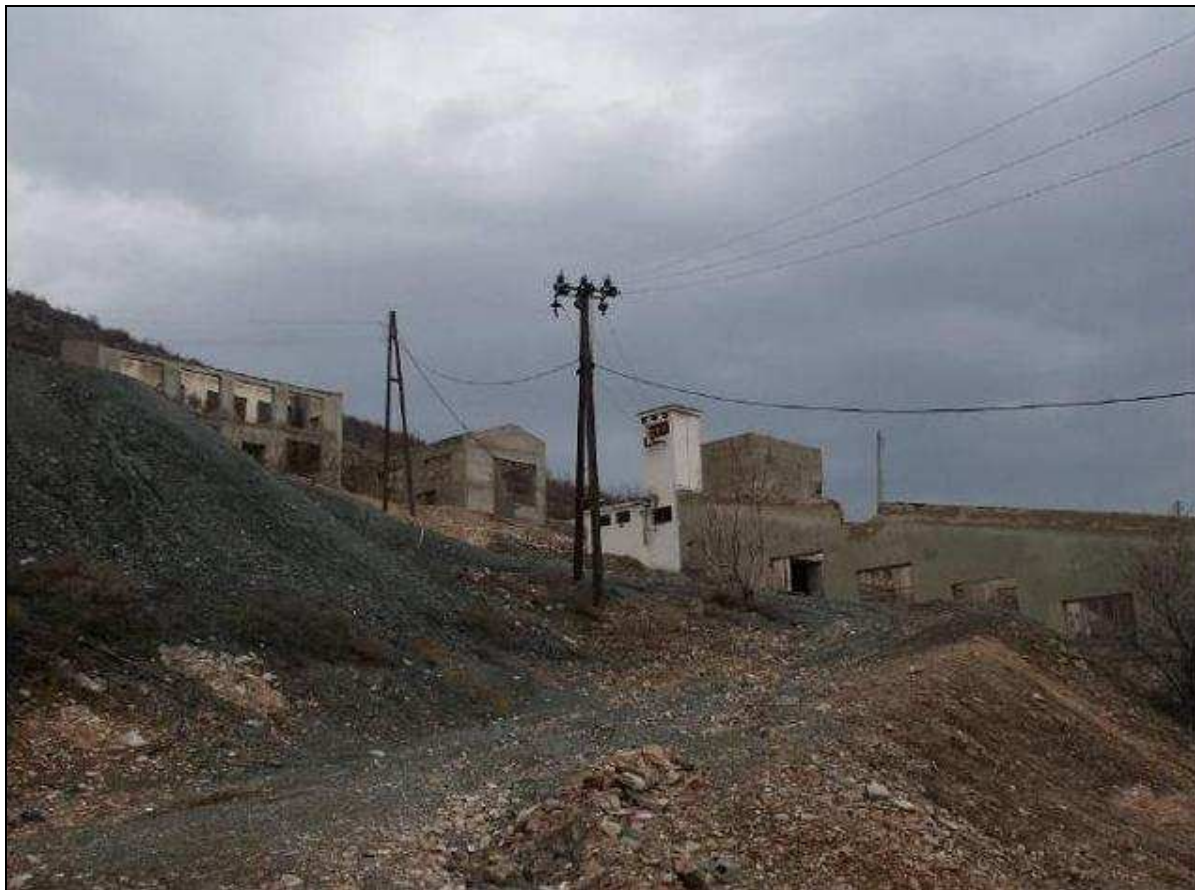
Photo 2.10 – Processing plant ruins
