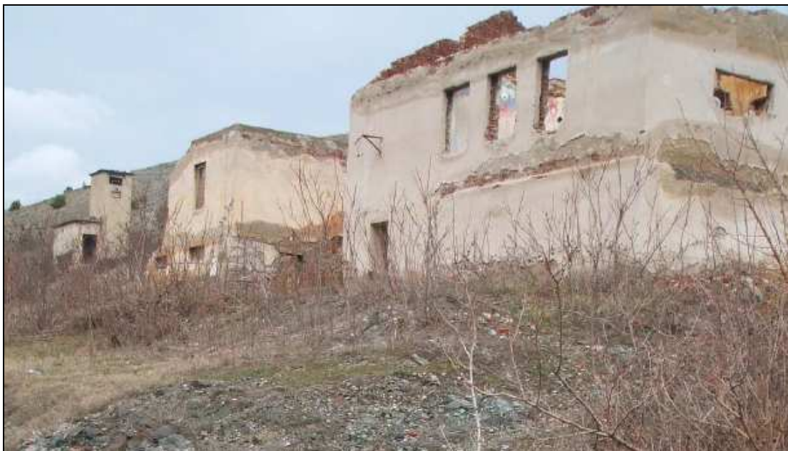
Photo 2.5 – Mine structures – old mining buildings
