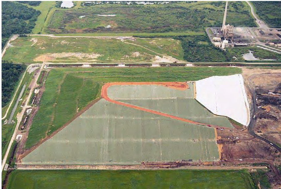
Figure 7-64: Exposed geomembranes cap used as final cover
