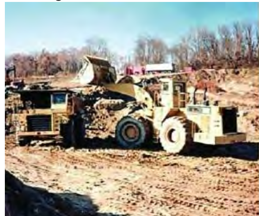
Figure 7-48: Compaction at the landfill and loading of soil cover material
