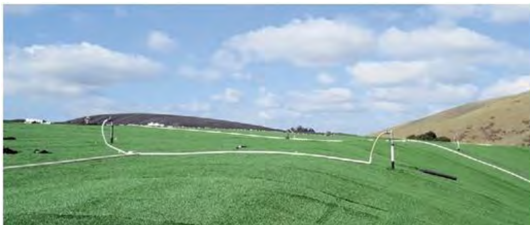
Figure 7-65: Closure Turf used as final cover
