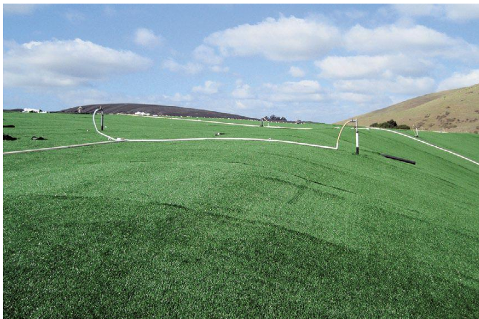
Figure 7-70: Closure Turf used as final cover
