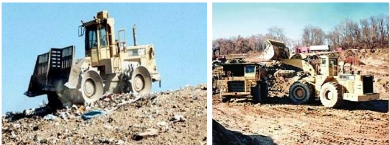
Figure 7-53: Compaction at the landfill and Loading of soil cover material
