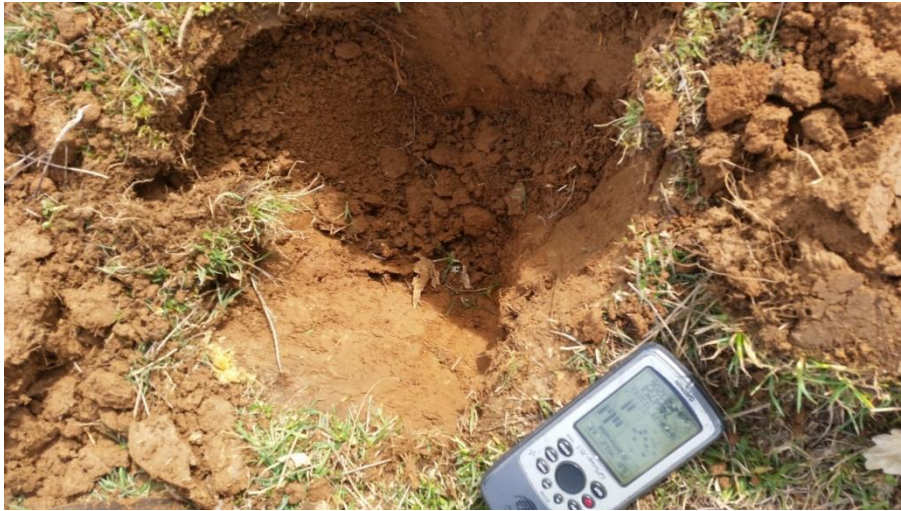
Figure 7-41: Investigative trench located in dusty clays
