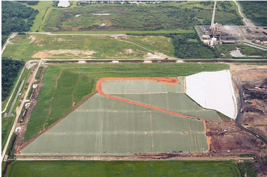
Figure 7-69: Exposed geomembranes cap used as final cover
