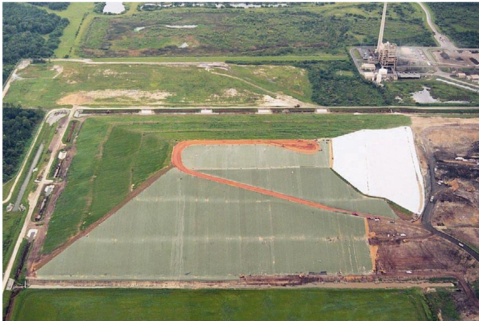
Figure 7-64: Exposed geomembranes cap used as final cover
