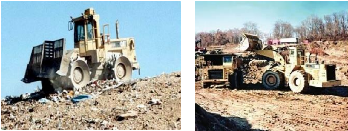
Figure 7-49: Compaction at the landfill and loading of soil cover material
