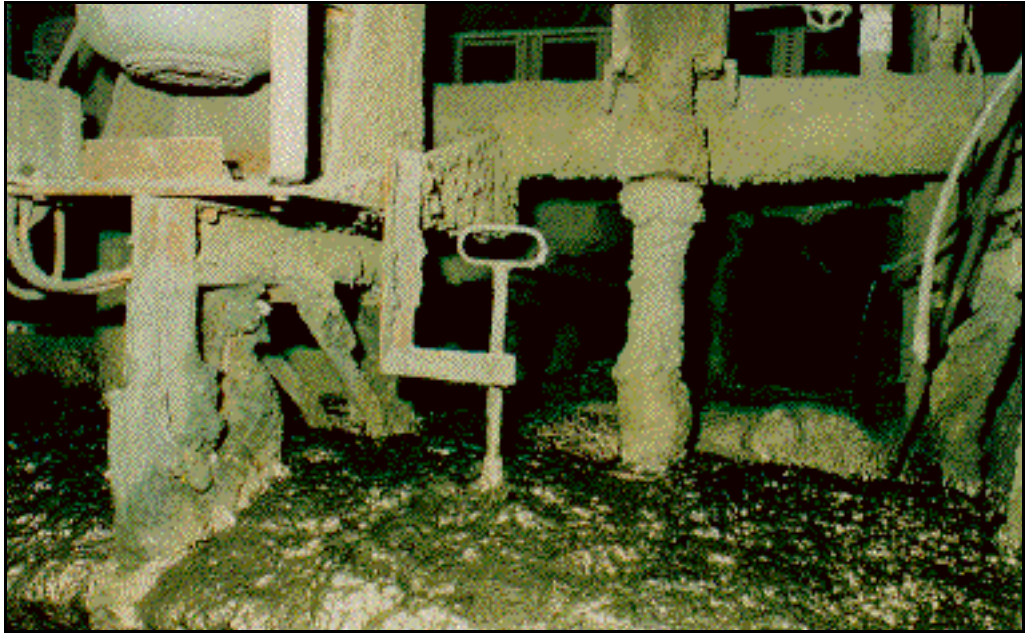
Flotation cell showing sodium ethyl xanthate addition point at right of centre.
