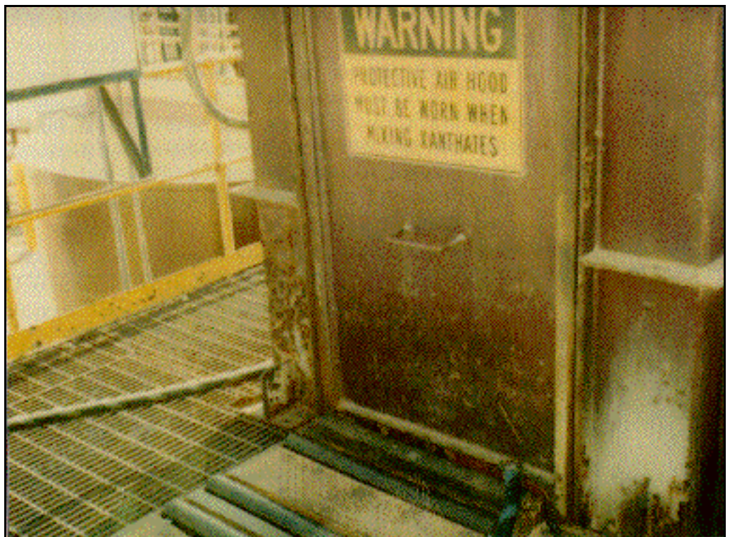
Door and rollers used for the emptying of drums into the mixing tank.
