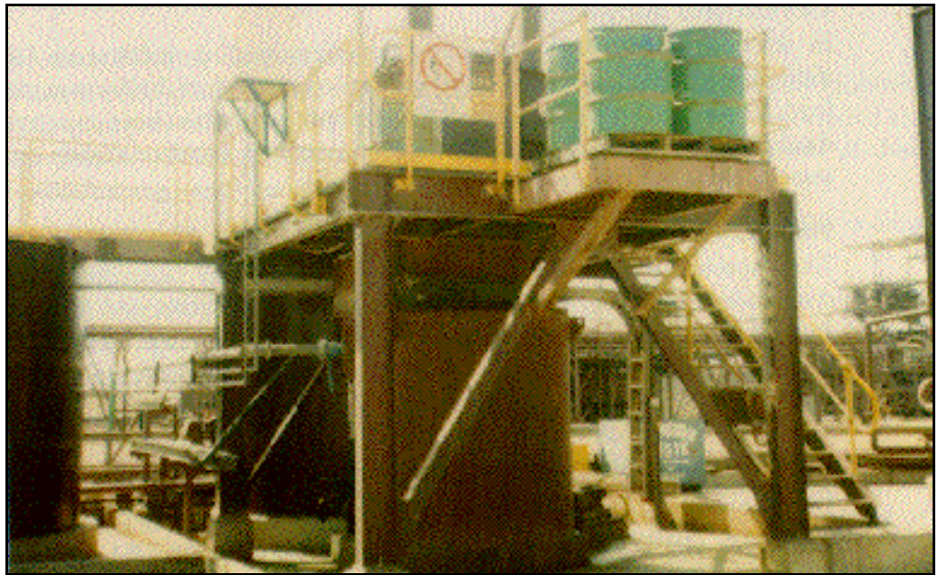
Ground level view showing mixing tank and drum storage area. Personal protective equipment stored in white box at left of picture.
